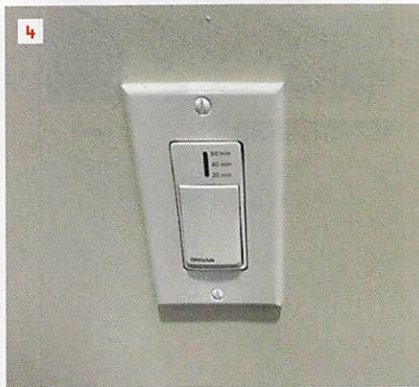
The Smart Wall Control (3) acts as a touch-screen interface for the ventilation system. In addition to allowing users to set the mode and monitor pollution levels, it allows manual control of the fan, functioning like a standard wall switch. In bathrooms, the author included ordinary timer switches for point-source control of exhaust fans (4).
