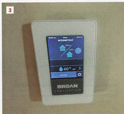
The Smart Wall Control (3) acts as a touch-screen interface for the ventilation system. In addition to allowing users to set the mode and monitor pollution levels, it allows manual control of the fan, functioning like a standard wall switch. In bathrooms, the author included ordinary timer switches for point-source control of exhaust fans (4).
